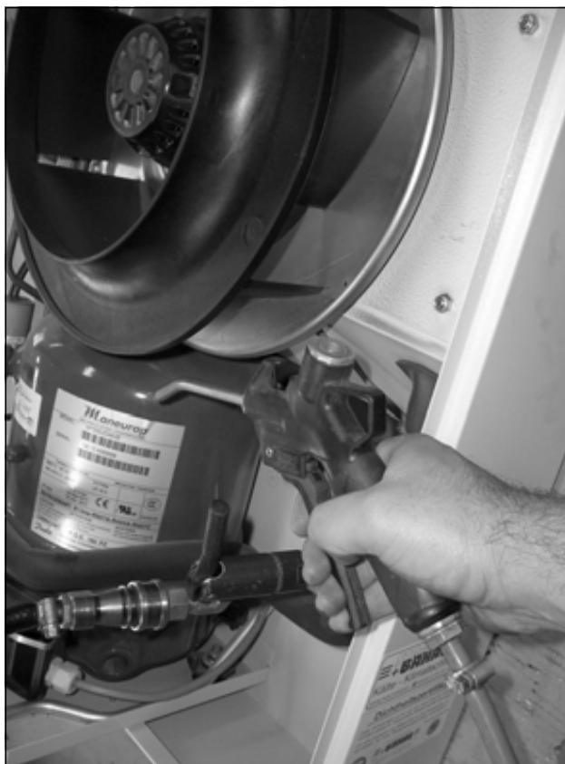
Fig. 57: Clean out the heat exchanger coil and compressor chamber using compressed air (2)
