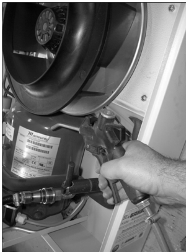
Fig. 81: Clean out the heat exchanger coil and compressor chamber using compressed air (3)
