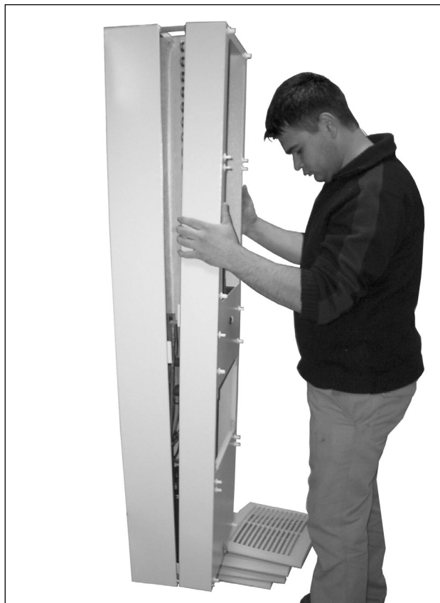
Fig. 76: Remove the cover
